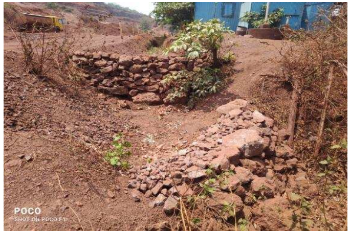
Photo-4: Showing Check weirs, Settling pond and Garland drain
