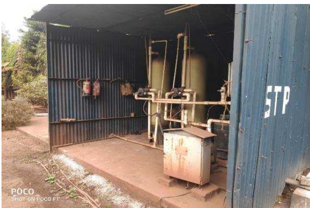
Photo-9: STP for treatment of Domestic Waste Water (Ultra Filtration Unit) & its utilization in green belt development
