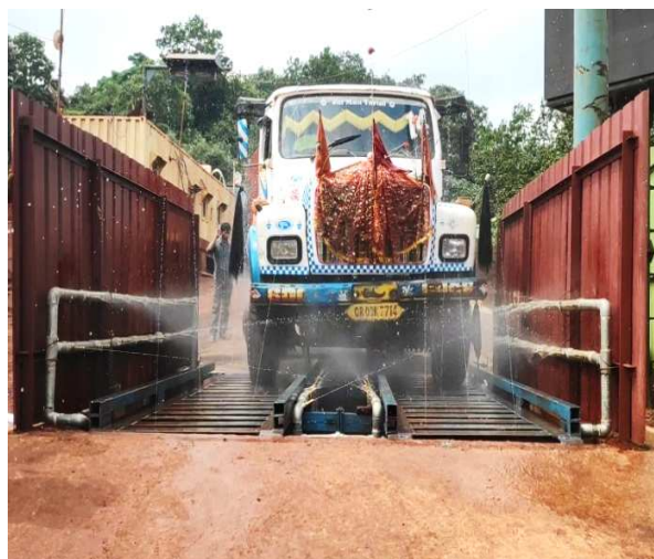
Photo-2: Truck Tire wash system
