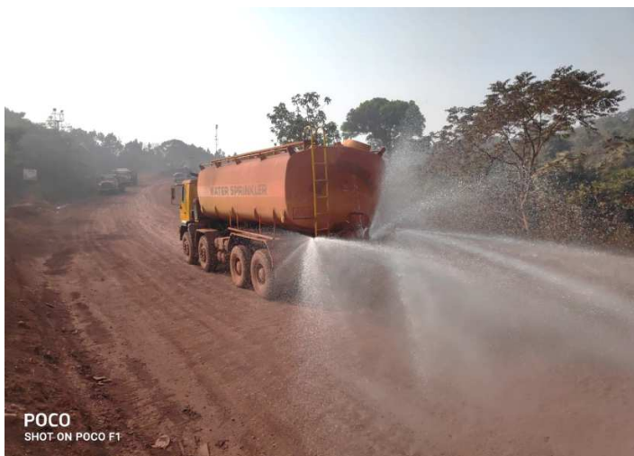
Photo-1: Mobile Water Tanker for dust suppression
